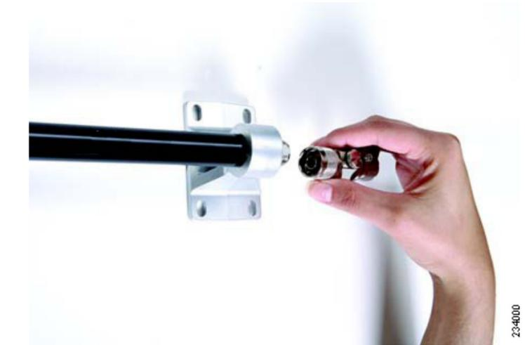
**STEP 2** Attach the untaped end of the antenna cable to the lightning protector.
